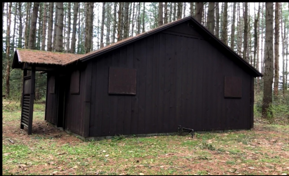
Comfort Station (In Camping Loop)
