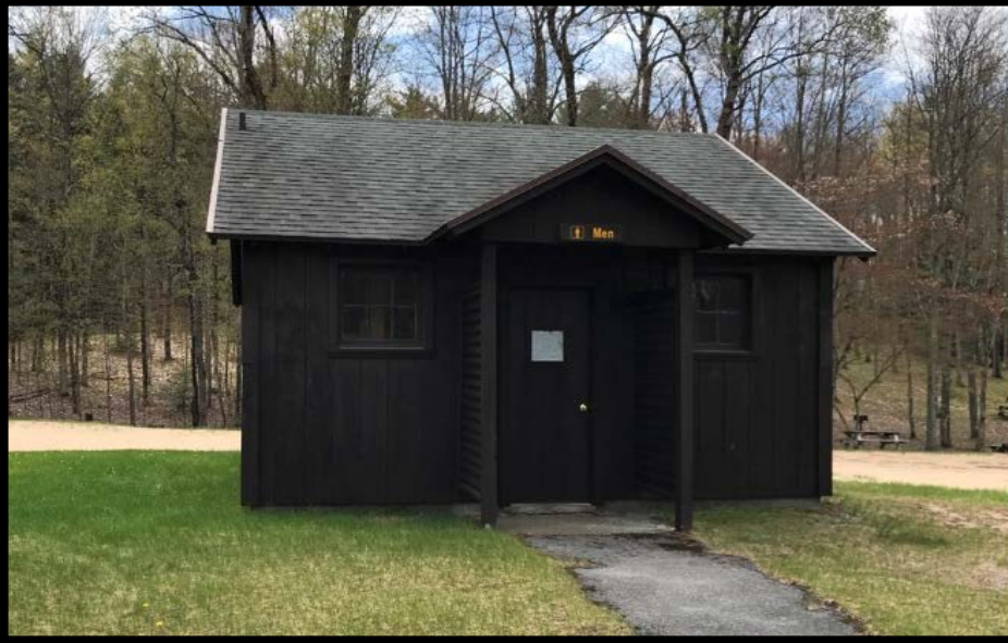
Comfort Station (South of Bathhouse)
