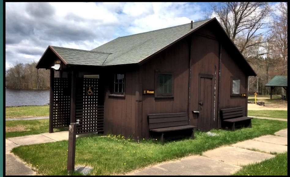
Comfort Station (North of Bathhouse)
